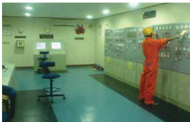
Figure 2. BROPSEEL© - Diesel Generators being synchronized after Black out by a Marine Engineering student.
